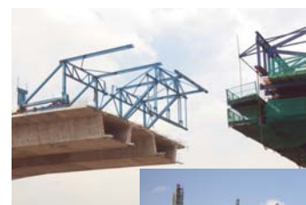
Chalifert High Speed Train Viaduct (France) Douce-Hydro's lifting and launching systems push the bridge deck. A total of 32 000 tons of deck was pushed over 3,2 km, allowing the construction of the high speed train rail tracks. 4 SA Hydraulic Cylinders dia. 530 mm, Stroke 70 mm 8 DA Hydraulic Cylinders 250 x 180, Stroke 250 mm 8 DA Hydraulic Cylinders 110 x 75, Stroke 1 000 mm 8 power packs + 4 sets of general mechanism
