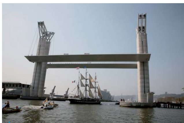
Mobile Bridge in Rouen, France 16 Hydraulic Cylinders DA 280 x 130, Stroke 1 000 mm +16 Hydraulic Cylinders DA 180 x 80, Stroke 1 000 mm
