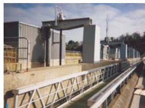
12 Servomotors Hydraulic Cylinders for La Rance tidal power station 670 x 170, Stroke 10 150 mm and 12 900 mm total rod length
