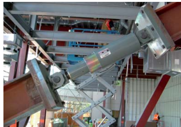
Amortecedores viscoelásticos ASR 1500-108 AH 200 kips, 4,0 pol. +/- Curso, a = 0,1 Viscous fluid dampers ASR 1500-108 AH 200 Kips, 4,0 in. +/- Stroke, a = 0.1
