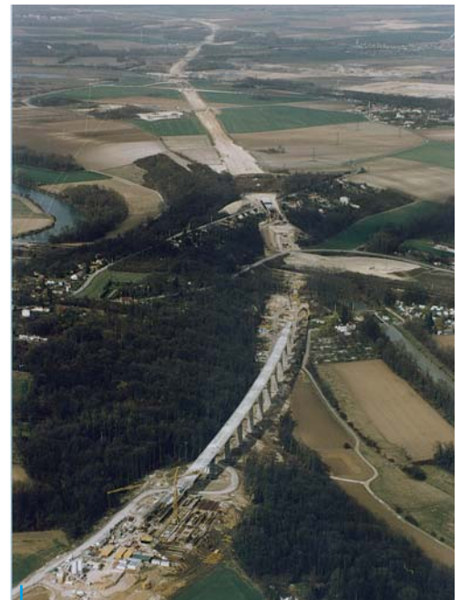
Chalifert High Speed Train Viaduct (France) Douce-Hydro's lifting and launching systems push the bridge deck. A total of 32 000 tons of deck was pushed over 3,2 km, allowing the construction of the high speed train rail tracks. 4 SA Hydraulic Cylinders dia. 530 mm, Stroke 70 mm 8 DA Hydraulic Cylinders 250 x 180, Stroke 250 mm 8 DA Hydraulic Cylinders 110 x 75, Stroke 1 000 mm 8 power packs + 4 sets of general mechanism
