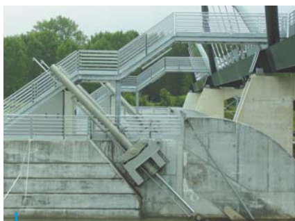
Dam of L'Isle Adam (France) 7 Hydraulic Cylinders DA 280 x 130, Stroke 5 600 mm
