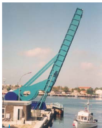
Mobile Bridge 2 Hydraulic Cylinders 250 x 200, Stroke 5 760 mm
